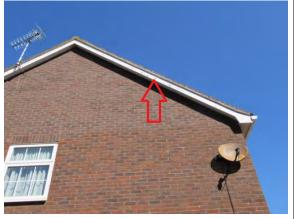
Poorly maintained bargeboards on the left side
